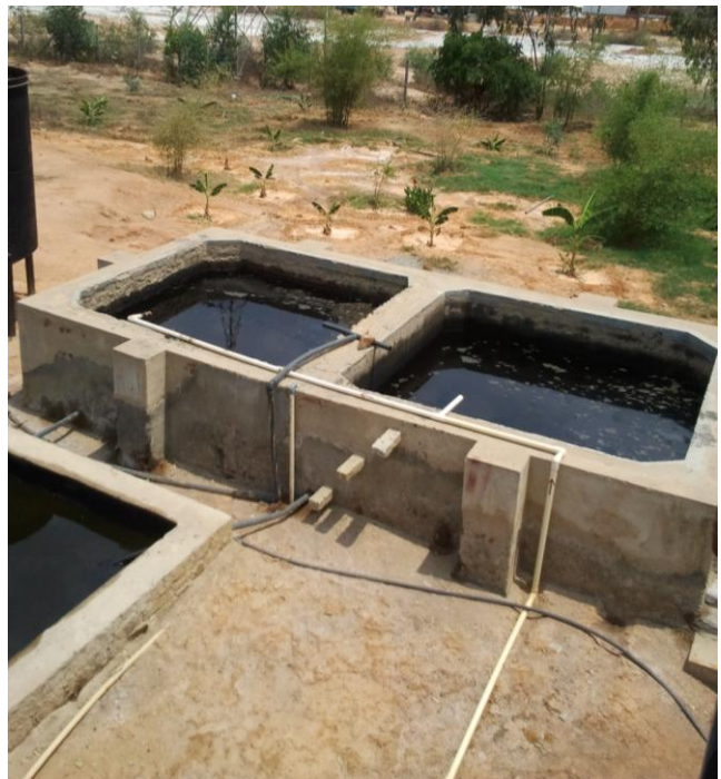
Fig 6: MEE concentrate storage tank
