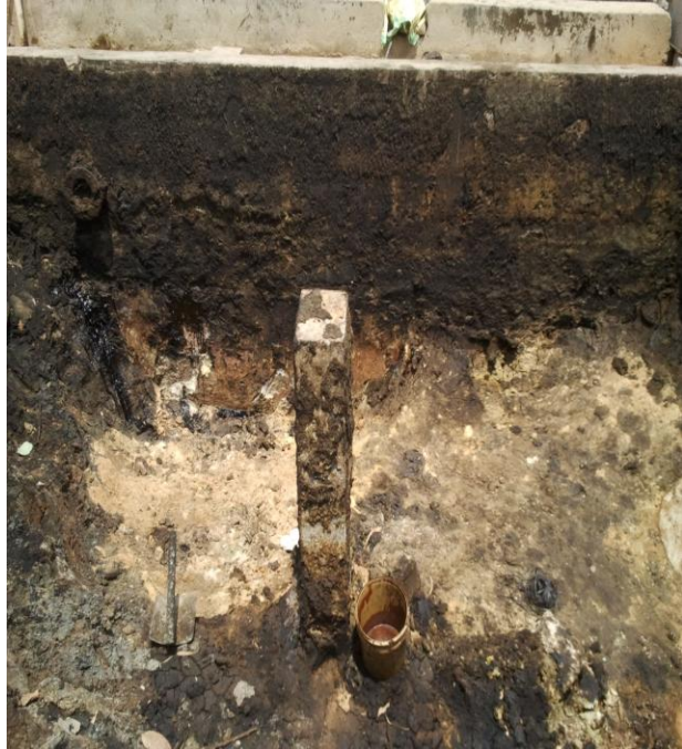
Fig 11: Sludge drying bed
