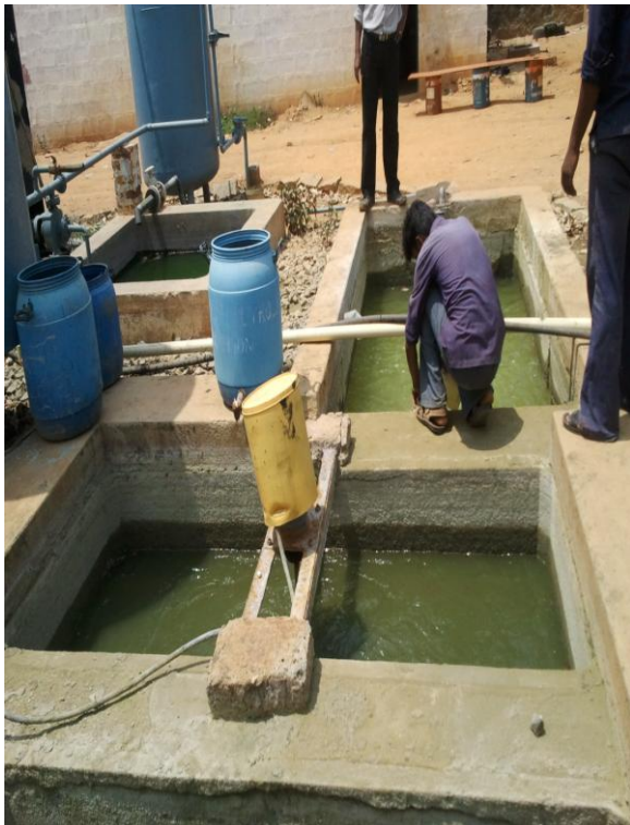
Fig. 9 - Low TDS effluent Settling tanks
