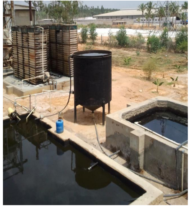
Fig 4: Conveyance of HighTDS effluent from storage tank to concentrate storage tank
