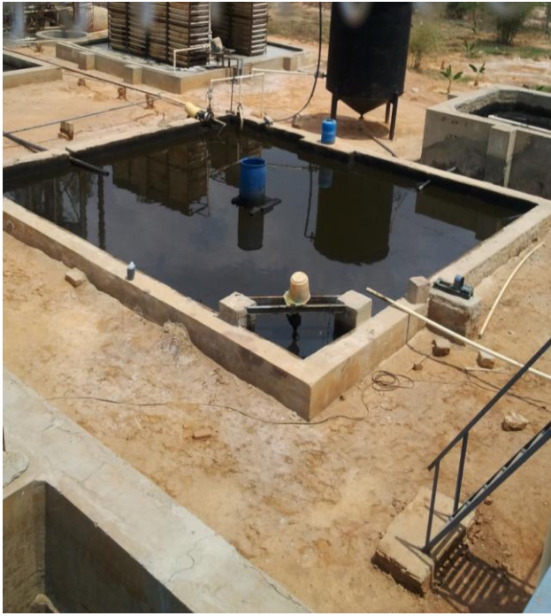
Fig. 3- High TDS Settling tank tank
