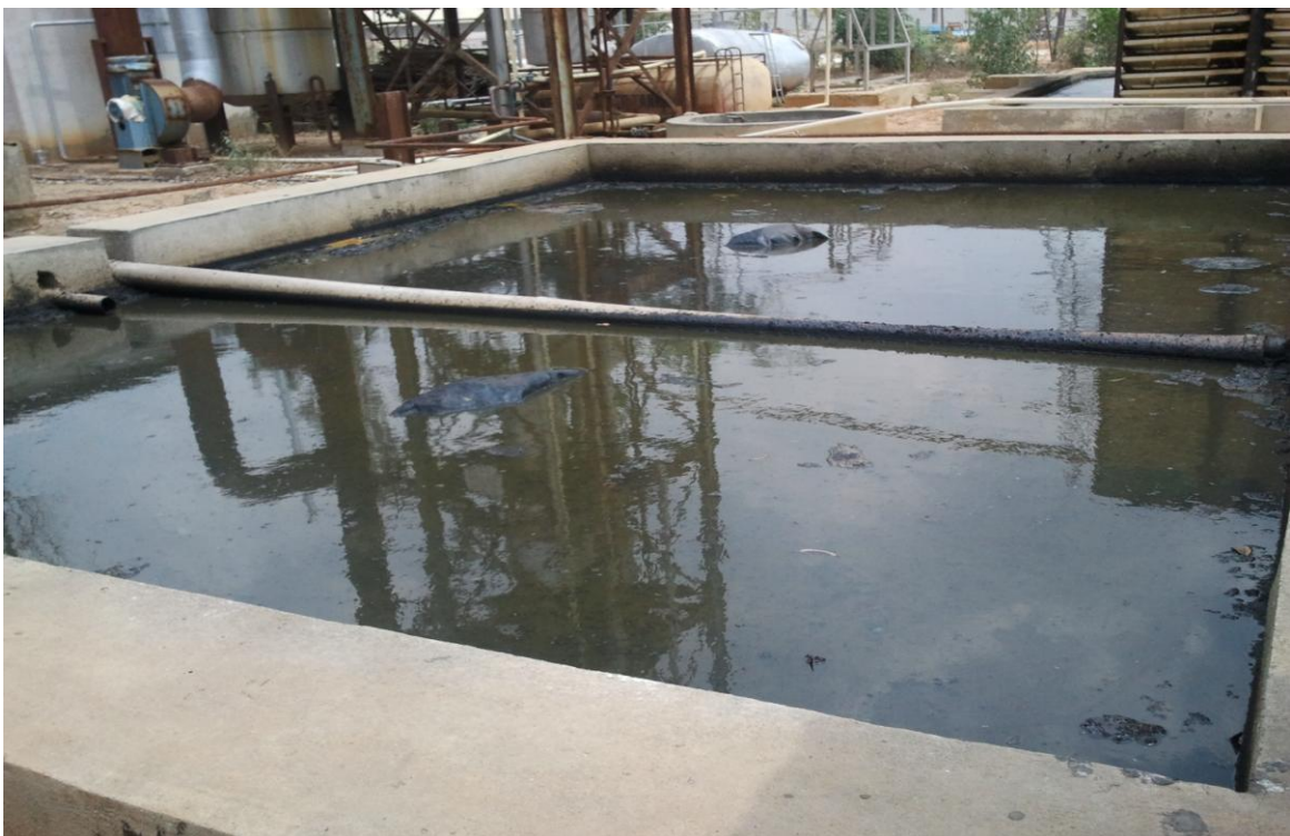
Fig 2: High TDS raw effluent storage tank
