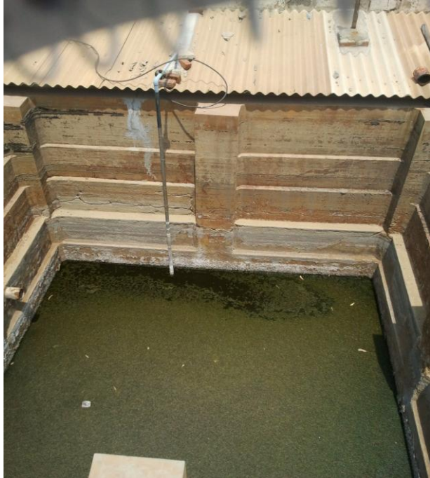
Fig 7: Low TDS effluent storage tank
