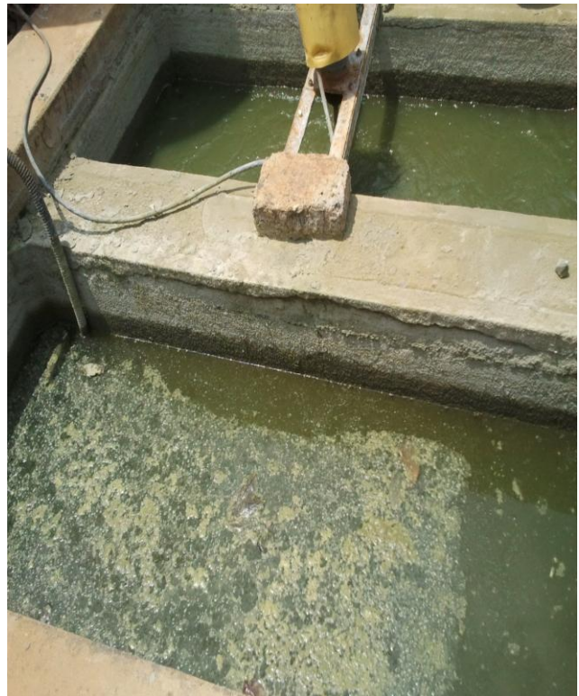
Fig. 9 - Low TDS effluent Settling tanks
